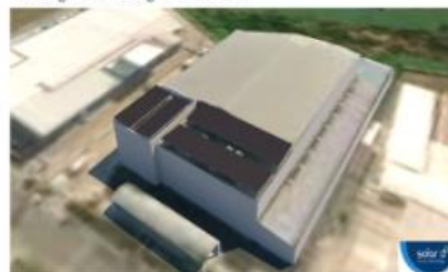
Proposed AYU1 Solar Roof to supply 100 Kw solar energy during day time.
